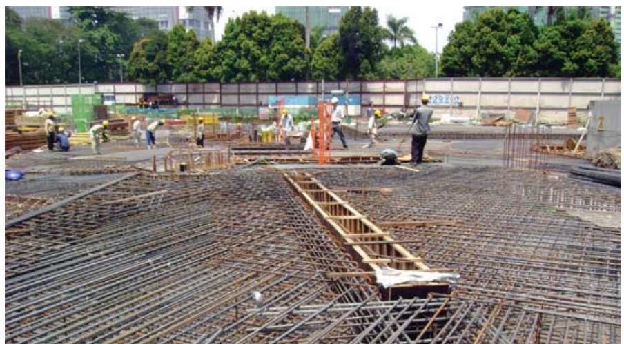
Construction project site
