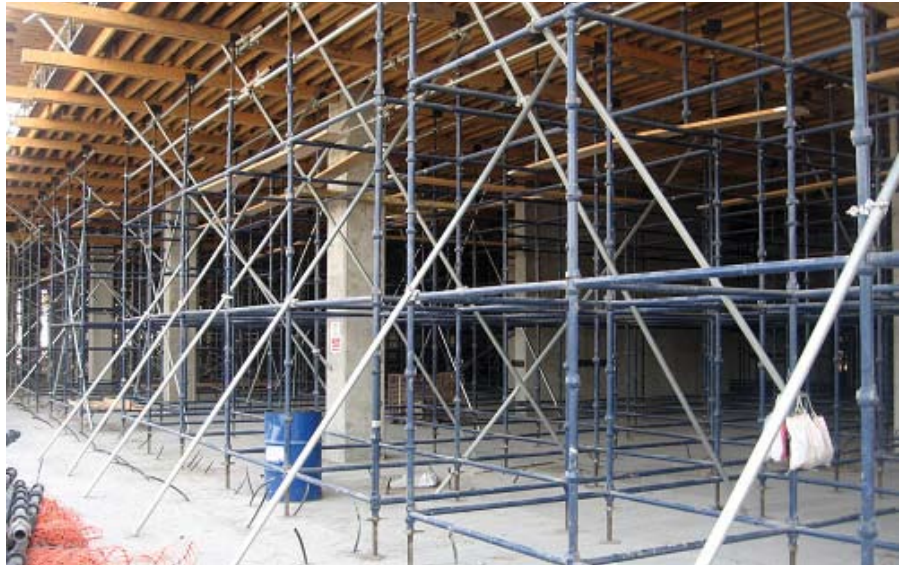
Partly completed building
